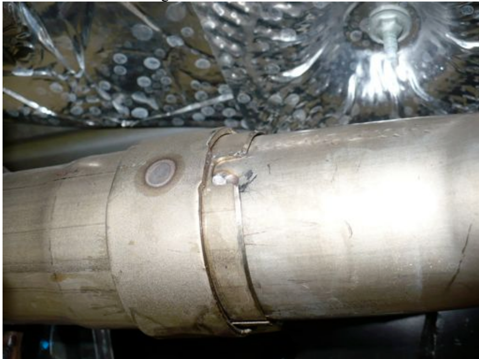
Image 3.2 with exhaust rivet removed
